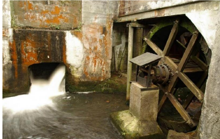
Fig. 1. General view of the power plant in Oliva (Poland) [20]
