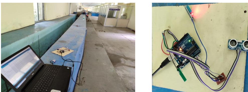
Figure 3 LoRa Transmitter setup At Canal Side
