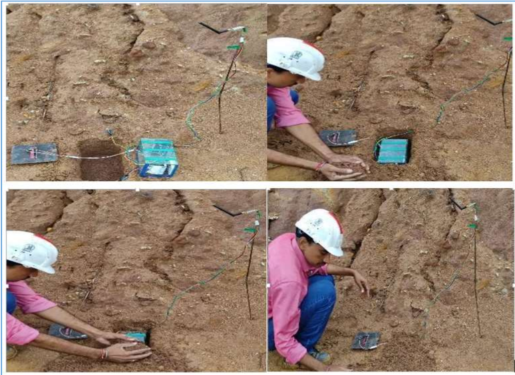
Figure. 7 Installation of sensor nodes on the slope benches
