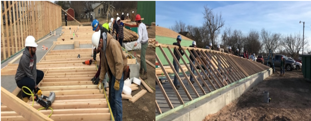
Figure 2. Students Framing and Raising Wall
